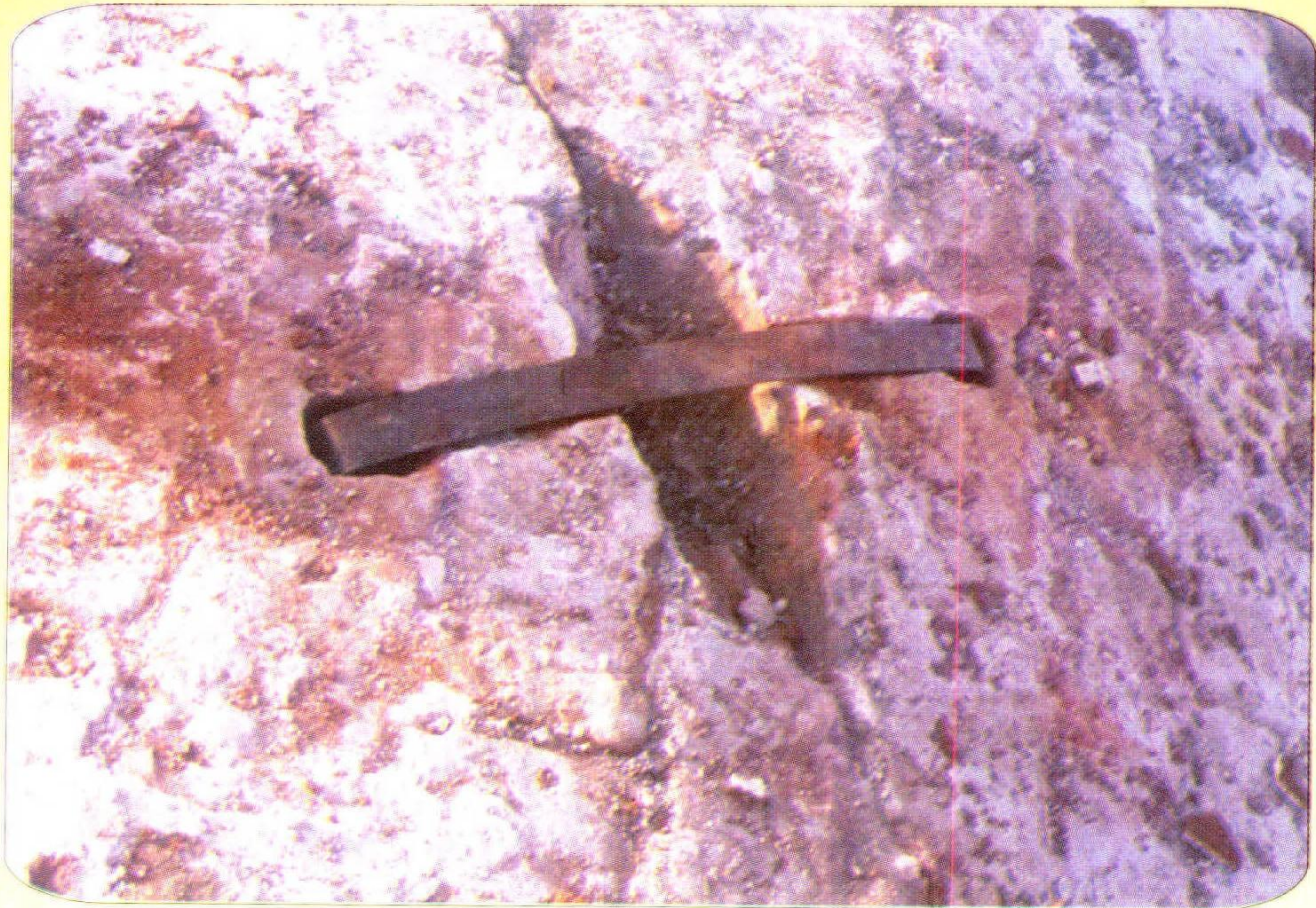
Crack in the arched portion being stitched with a copper clip.
