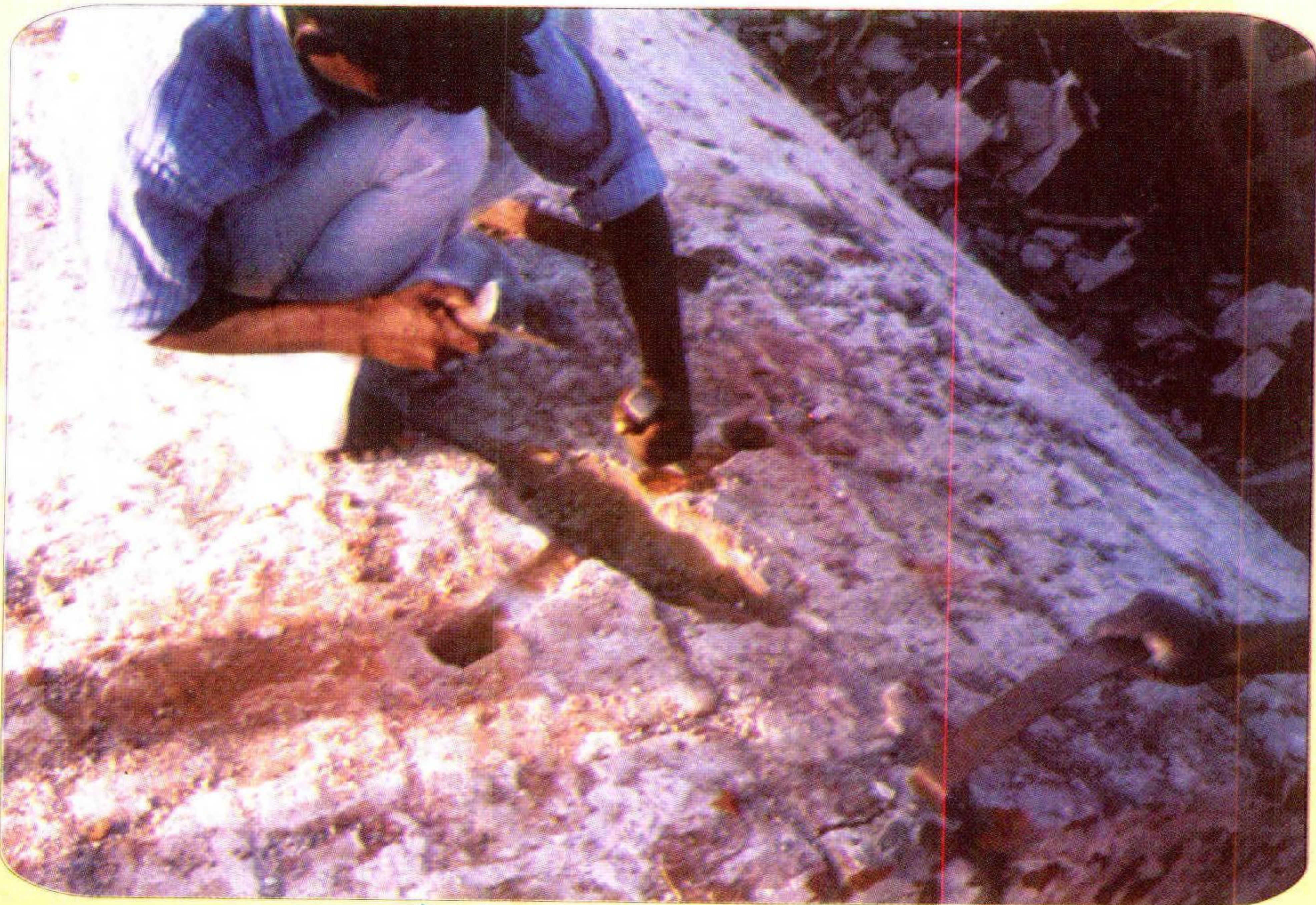
Making a groove to place the copper clip before pouring lead to stitch the cracked roof.
